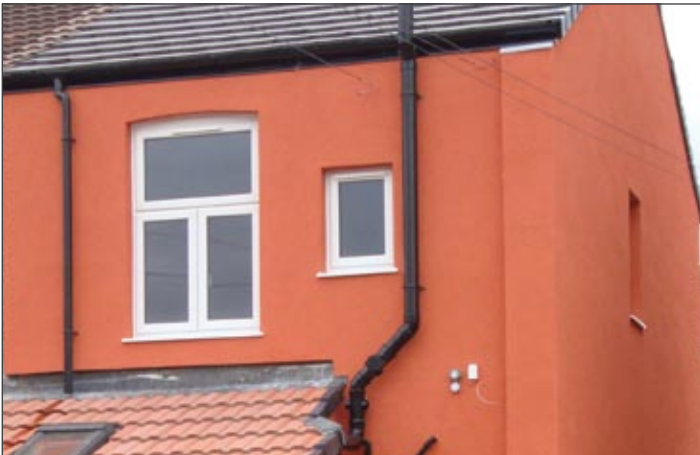
Photograph of rear elevation and gable after refurbishment using Structherm External Wall Insulation and through coloured render.
